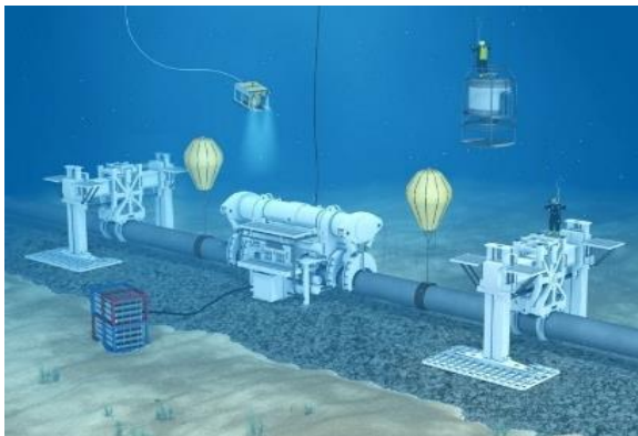
Fig. 5. Cofferdam welding
